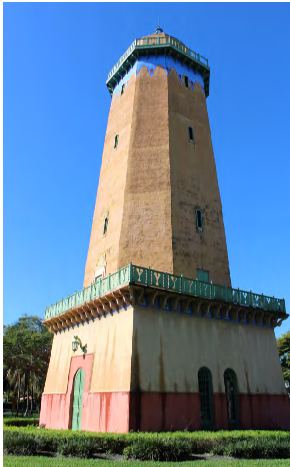
Alhambra Water Tower - Built in 1924 to conceal a steel water tank
