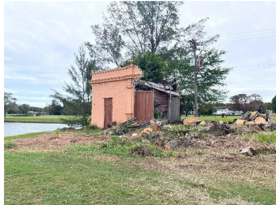
Current conditions- Gondola Building -north facade (2024)
