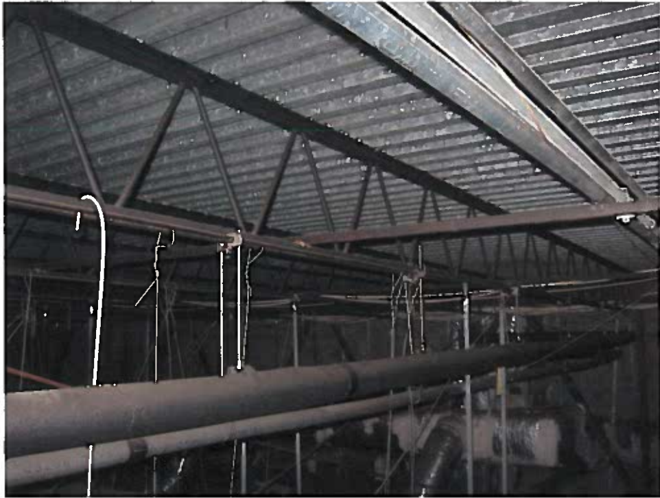
Picture 4: Existing Steel Roof Structure
