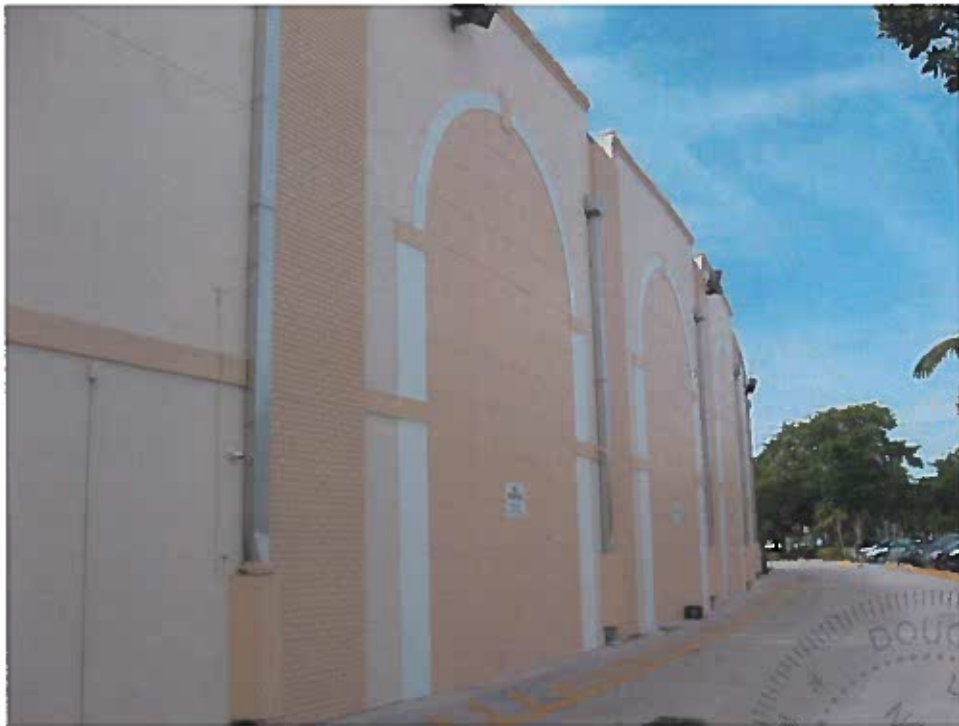
Picture 5: Existing Bearing Masonry Walls
