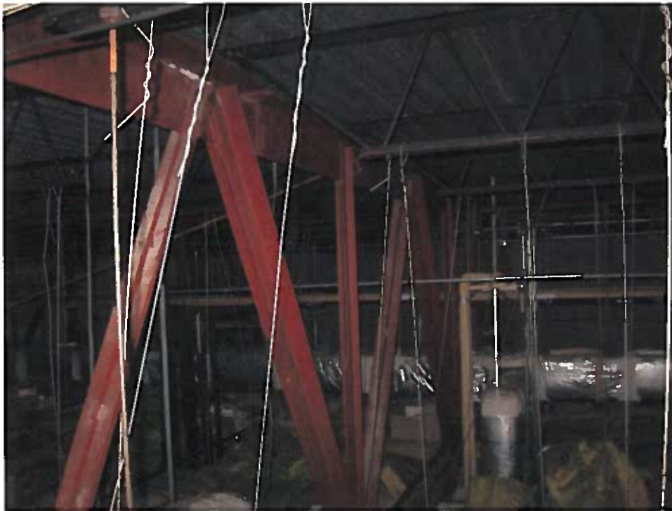
Picture 3: Existing Steel Roof Structure
