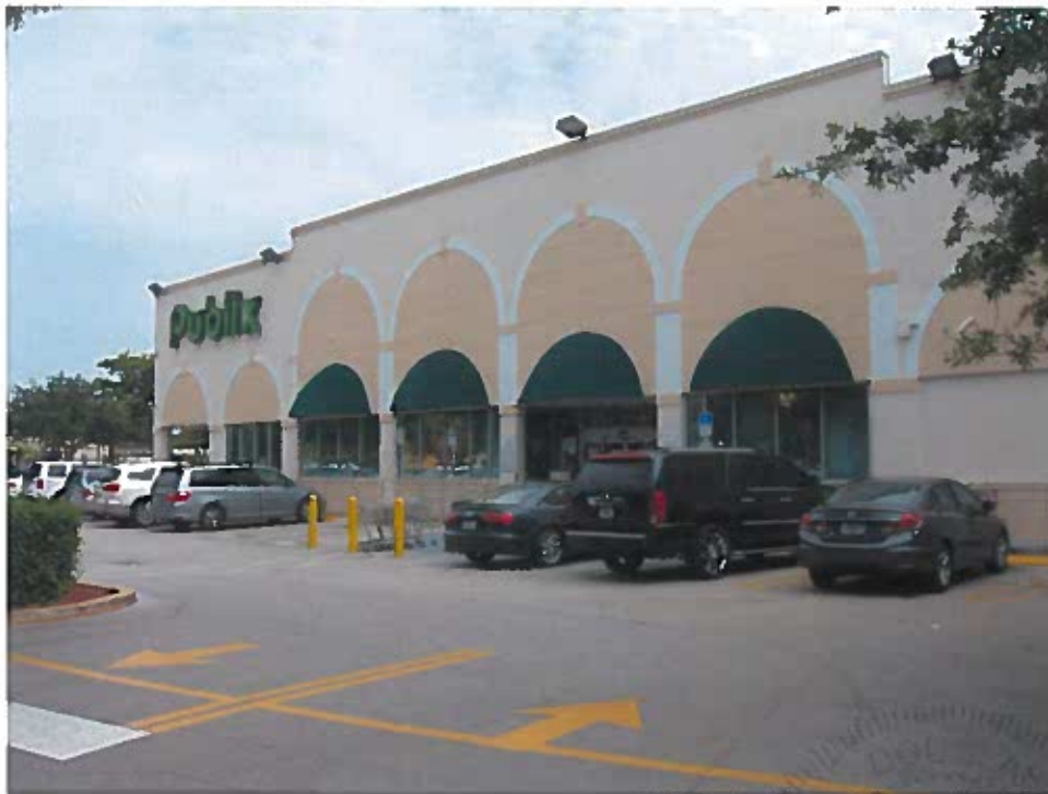
Picture 1: Front of Existing Building
