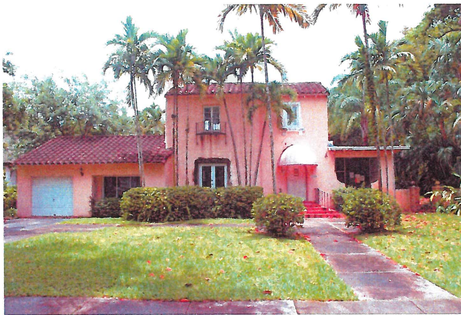
Front Façade Photo 2012
