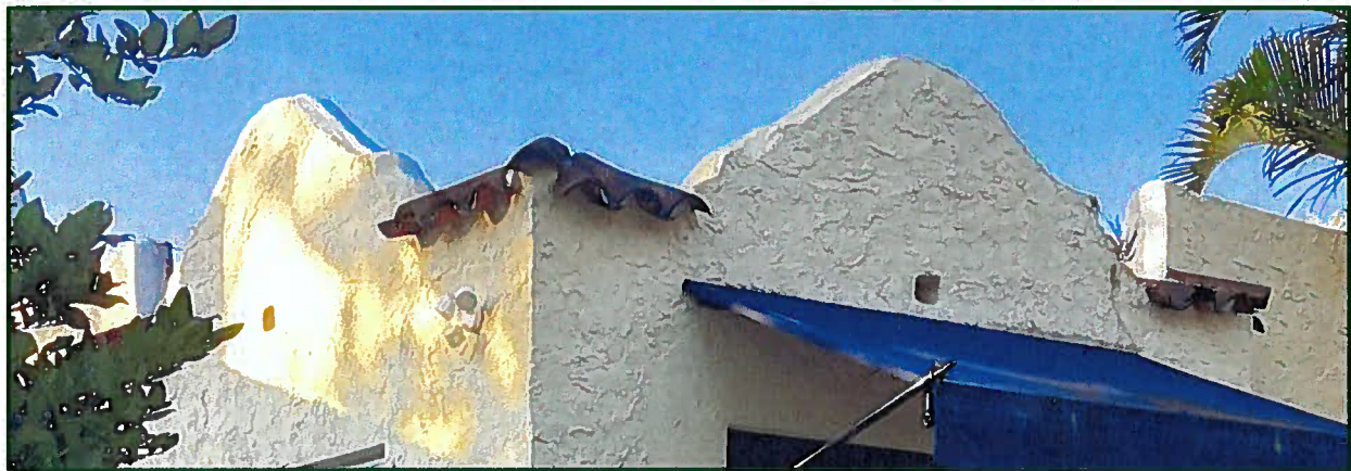
Figures 11: Notable Features, 2024 Chimney with Geometric Cap [top] Front Entry Porch Parapet Ensemble [bottom]
