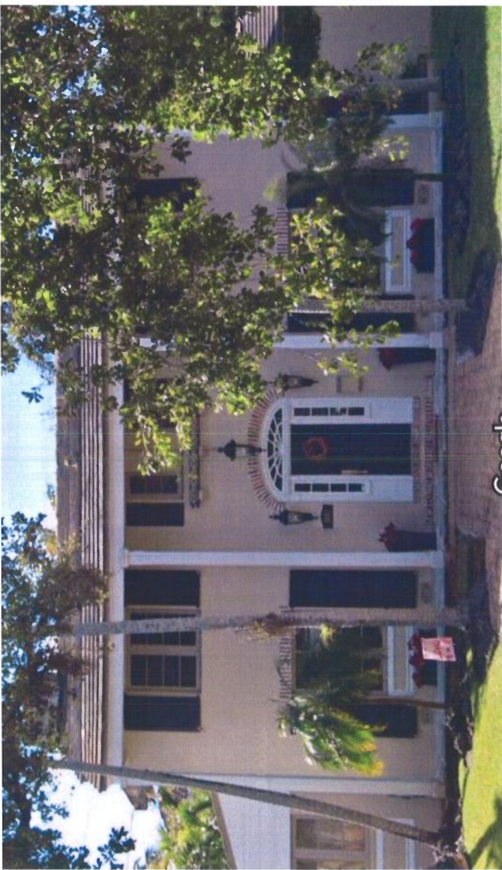
3402 Toledo St has the same brick steps, fanlight, sidelight, and proportions as 649 Palmarito Ct the same door and window details, layout, and proportions as 649 Palmarito Ct
