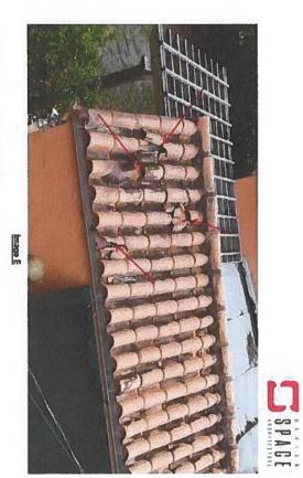
This image shows several "S Tile" rooting tiles either broken or damaged.
