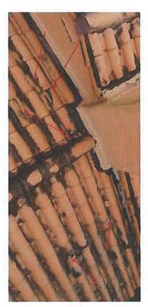
This image shows several "S Tile" rooting tiles either broken or damaged.
