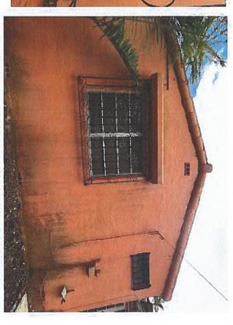
Openings on rear wall changed extensively. Openings cannot be reversed without extensive concrete work and cost.
