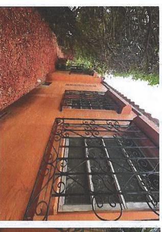
Openings on East wall changed over renovations. Openings cannot be reversed without extensive concrete work and cost.
