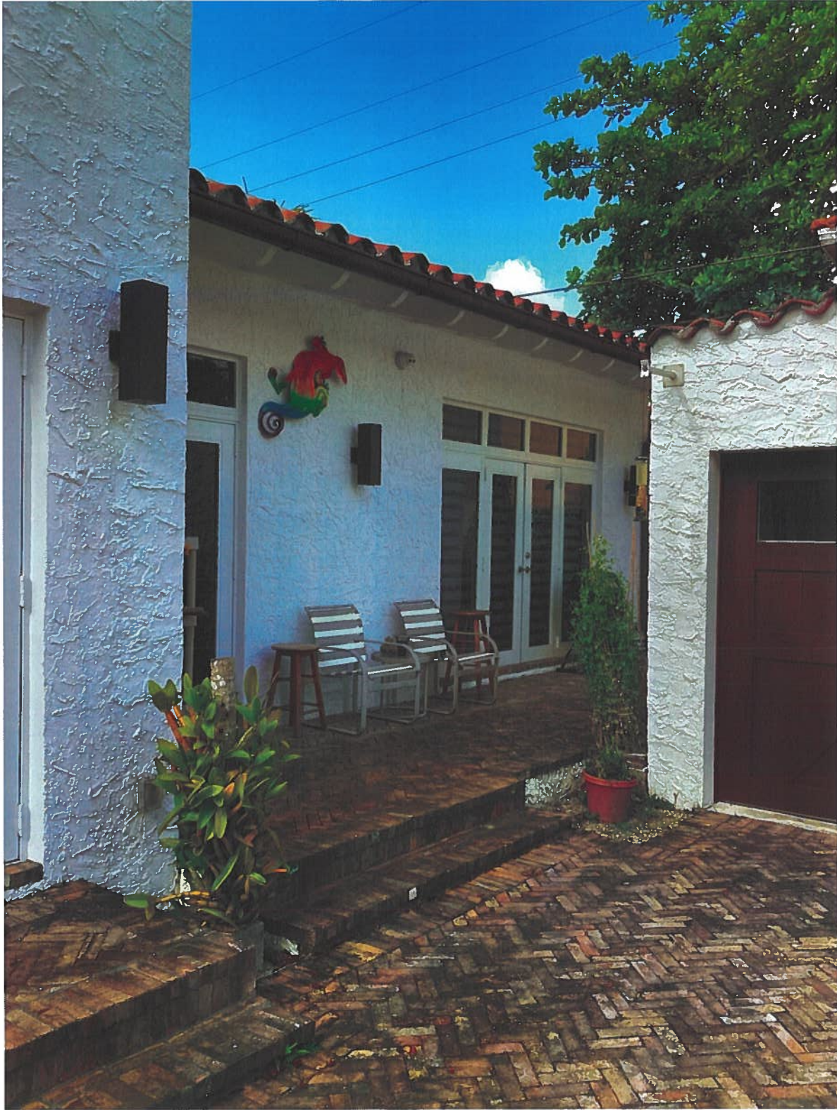
Remove the covered porch addition from the 1950s and replace it with a new Mediterranean Revival style addition - 2
