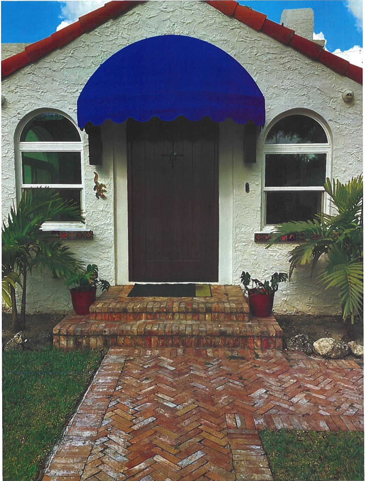
Recessed arched windows with projecting masonry lintels
