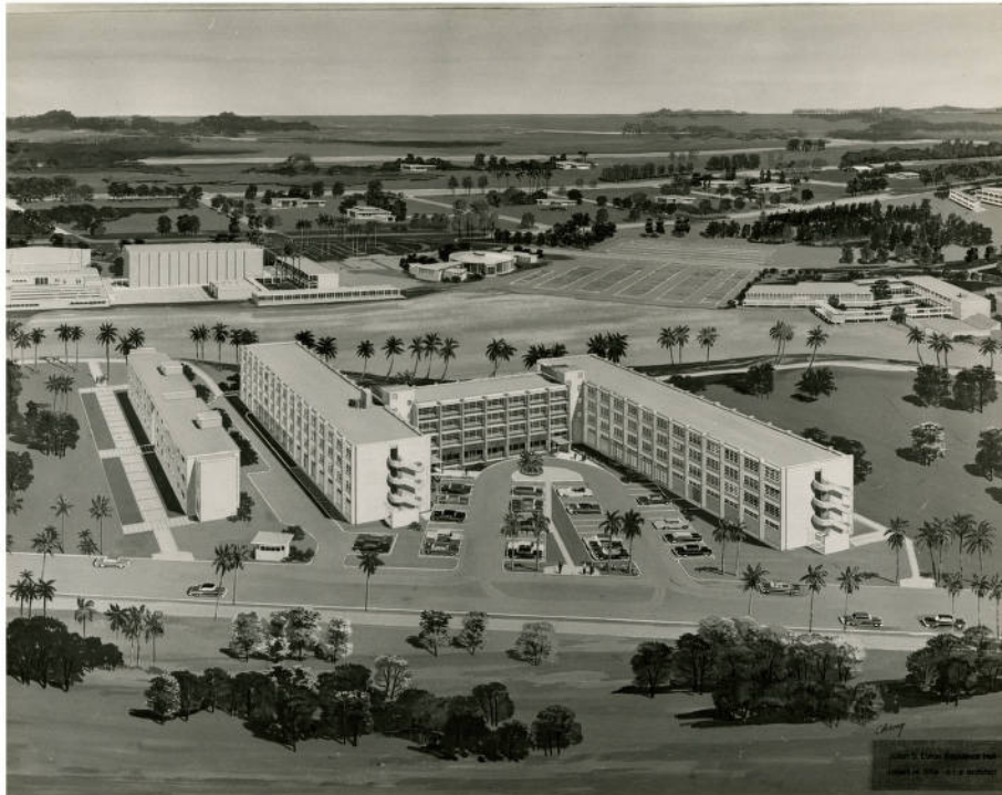
Architectural model demonstrating how Eaton's expansive H-plan maximizes surface area and exposure to the outdoors
