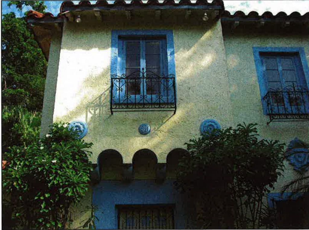
Bay window at Front Elevation- South
