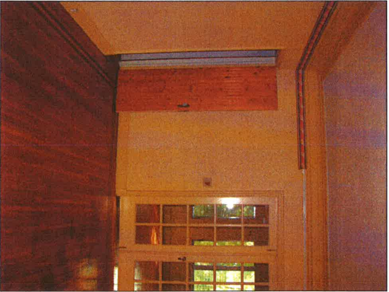
Ceiling plaster crown moulding at Master bedroom
