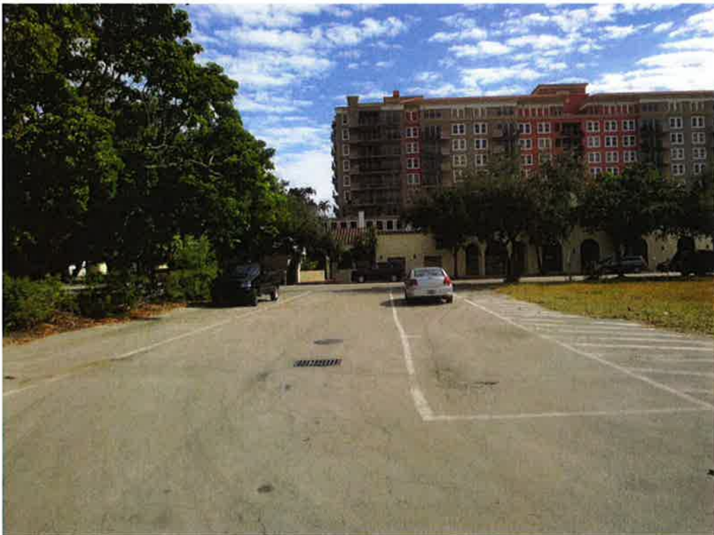
Photo 10: View of the existing E-W alley –looking east from site.
