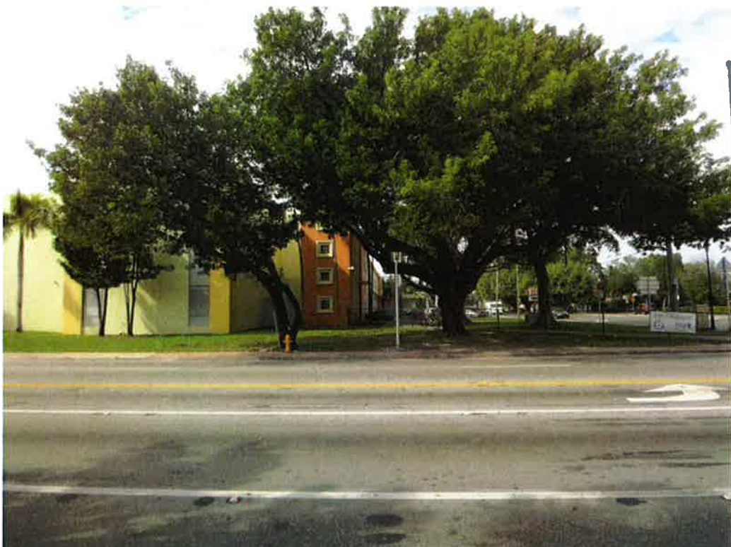
Photo 6: View of the existing Coral Gables High School – across Le Jeune looking west from site.
