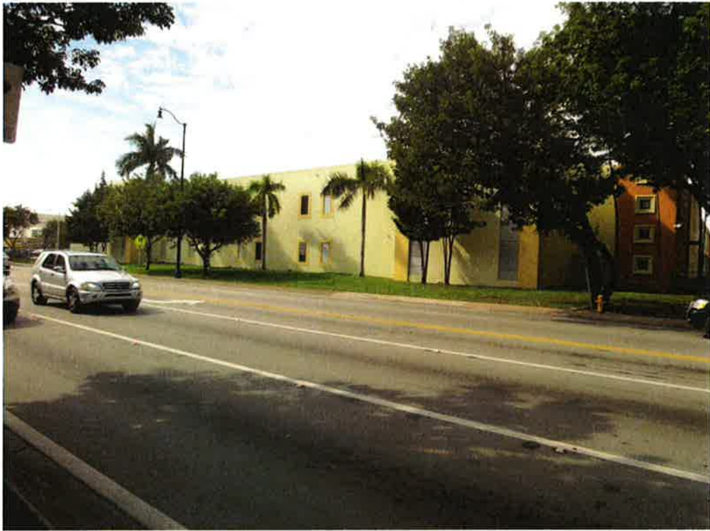
Photo 7: View of the existing Coral Gables High School – across Le Jeune looking southwest from site.
