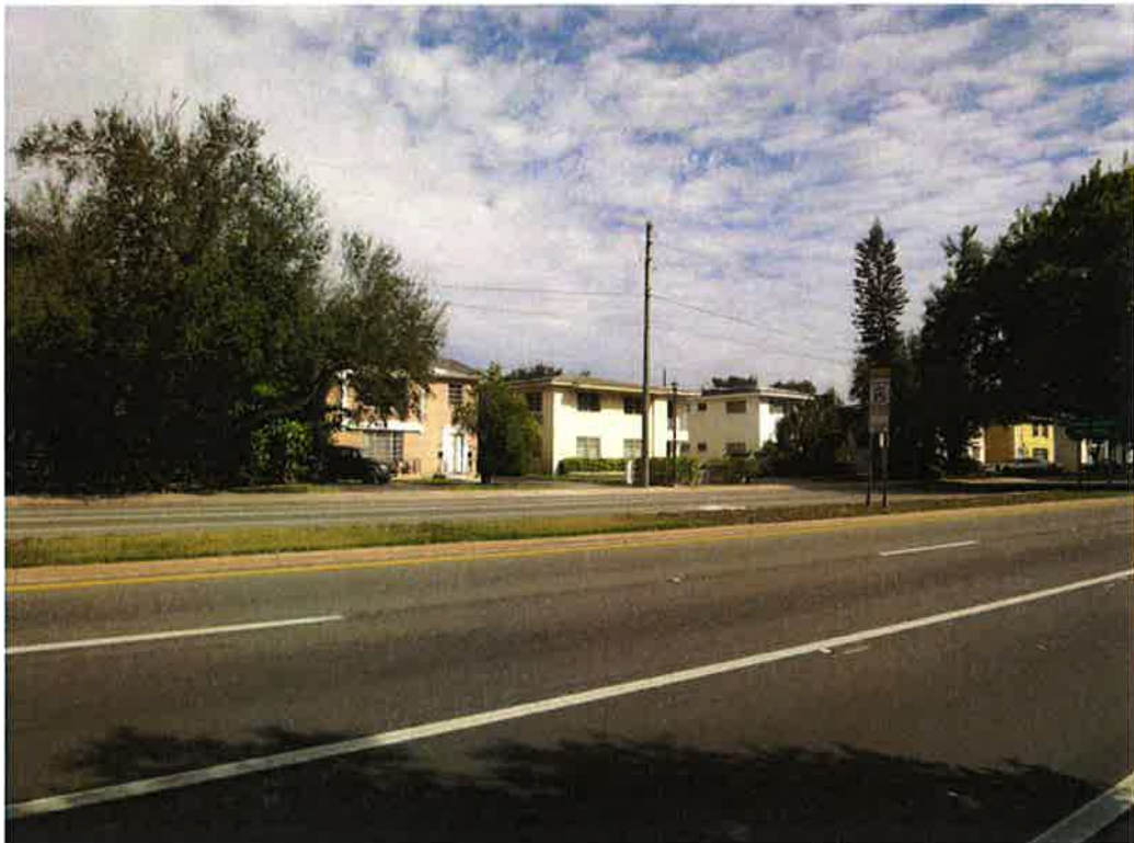
Photo 8: View of the existing apartments – across Bird Rd looking northeast from site
